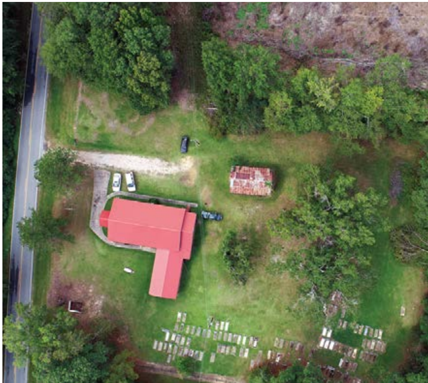
Researchers at Penn's Center for the Preservation of Civil Rights Sites and Tuskegee University are collaborating on stabilizing the structure and developing an interpretation plan for the historic Armstrong School.
